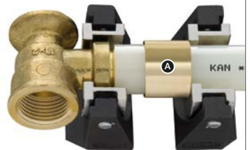
Installation of brass wallplate elbows
